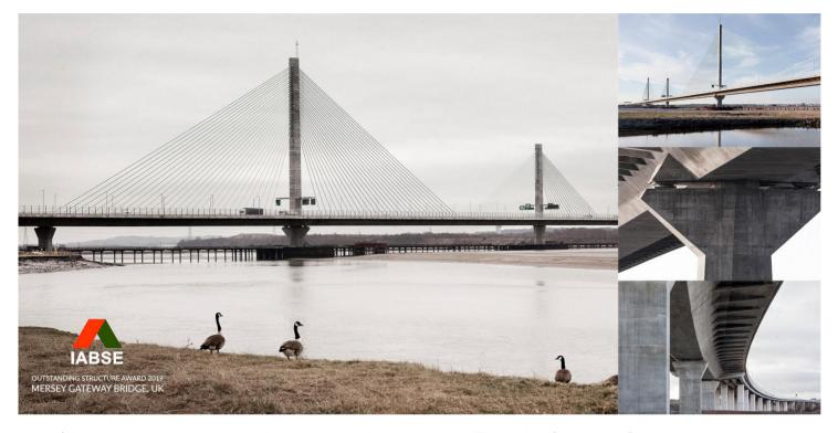
Mersey's bridge is a continuous structure 2248 m long without intermediate expansion joints. The central part (around 1000 m) is a four spans cable stayed structure.
